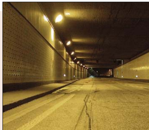
Boring tunnel is a gold mine for ecologists.
